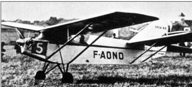
Below: F-AONO was an SFCA-built tandem-wing single-seat Taupin. With STOL performance it was appropriately named after a French jumping beetle! (all via JM Collection)
