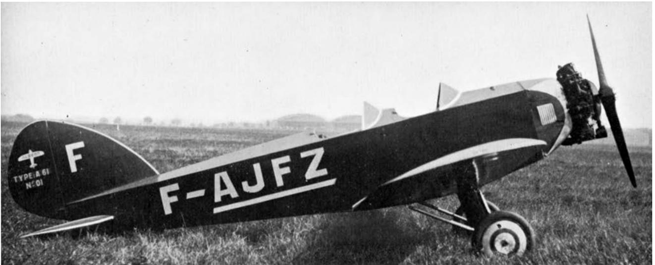
**Above:** F-AJFZ was the Albert A.61 two-seat open-cockpit tourer fitted with a 95 hp Salmson engine. The remains of this aircraft were discovered in 1999 and restoration continues. (via JM Collection)
