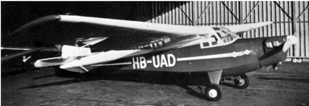
**Left:** This Praga E-114 was built as a 114M c/n 122 and went to France as F-BCSQ initially. Sold to Switzerland in 1952 it became HB-UAD and was converted from Mikron to 65hp Continental power and registered as an E-114C.
