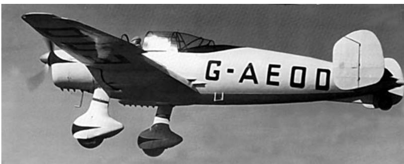
**Above:** As the fly-past continues with flaps lowered the R.S.1 shows the fixed step behind the wing root from which the crew gained access to the walkway and cockpit - quite a steep climb with the long fixed undercarriage raising the front well clear of the ground. The unusually-shaped vertical tail surfaces are also clearly visible, these were fabric-covered, and the un-trimmed balanced rudder line stands out well. (Flight via JM Collection)
