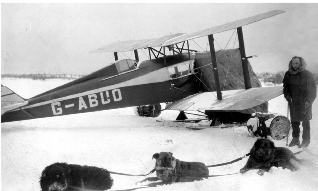
**Above:** After arriving in Canada in 1932, c/n 4000 retained its British registration during trials. Here it still has the open pilot's cockpit during tests on Fairchild floats.
