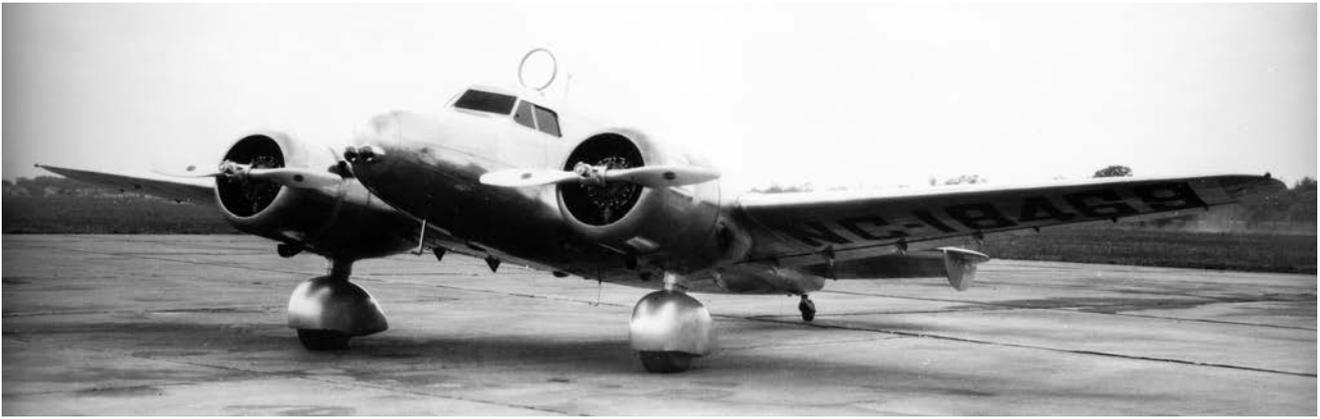
**Above and Right:** Two early views of msn 5 when still registered as NC18469. The DF loop above the cockpit and the twin landing lights in the nose are features of this airframe. (John Wegg collection)
