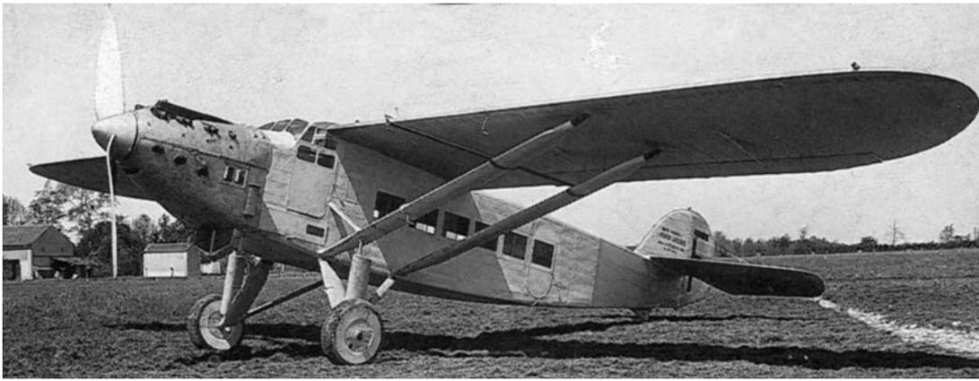
**Left:** Latécoère 28/1 prototype F-AJHS (500hp Hispano-Suiza 12Hbr twelve-cylinder water-cooled vee) eight passenger airliner. Used in some numbers by Air France and South American airlines, it was also available in military and floatplane configurations.
