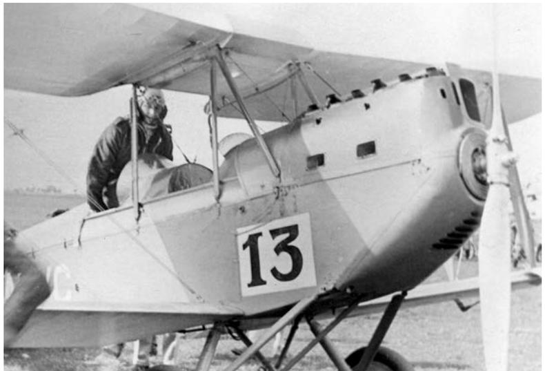
**Right:** While a number of engine options can be considered as standard, one that seems to have been applied rarely was the 130 hp DH Gipsy Major 6-cyl inverted seen in this example. (via JM Collection)
