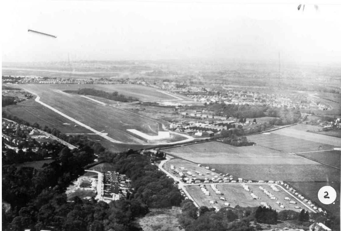
On approach from the east over Hoburne Caravan Park.
