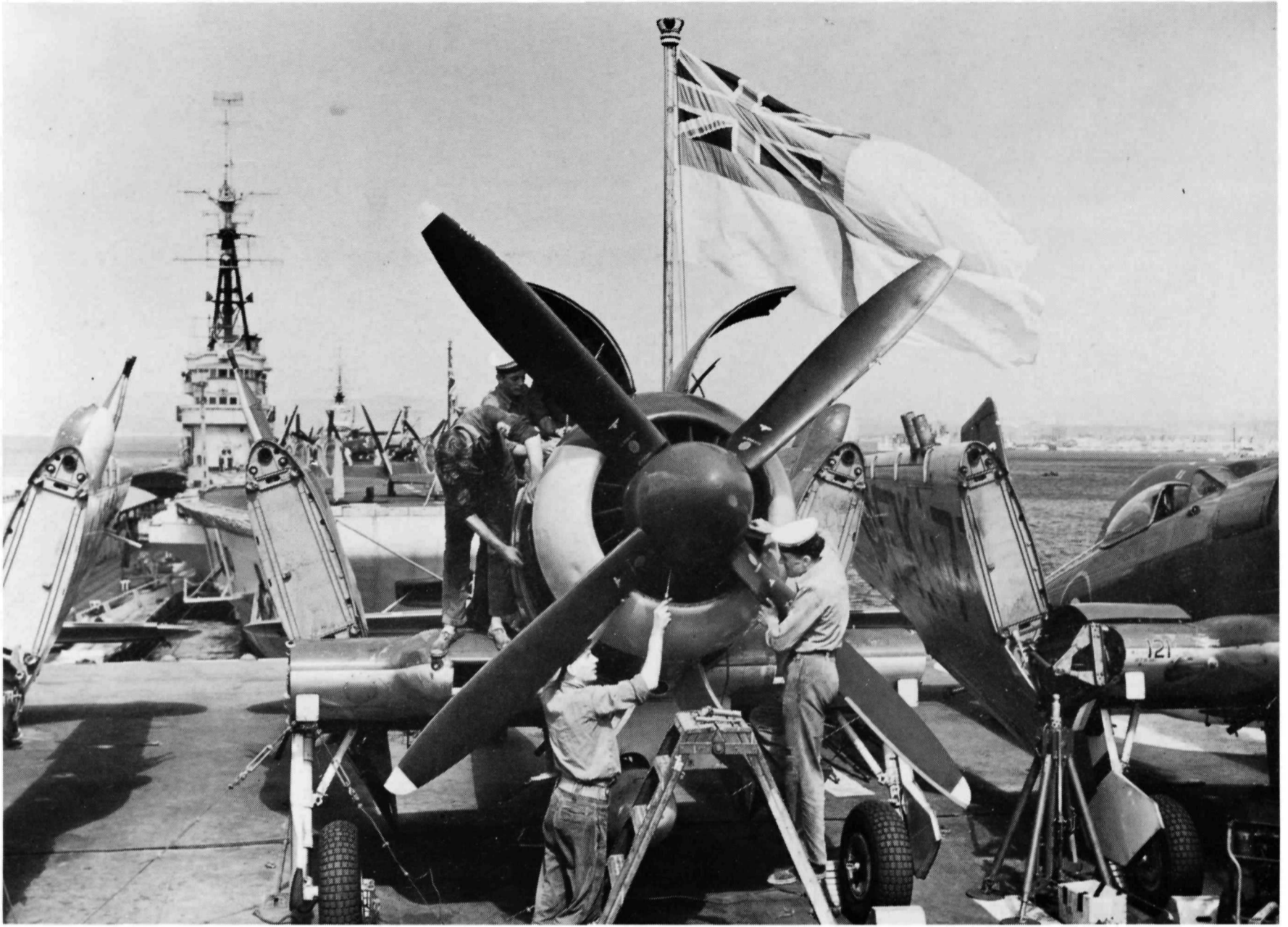
Servicing a Firebrand on the stern of Implacable at Gibraltar
