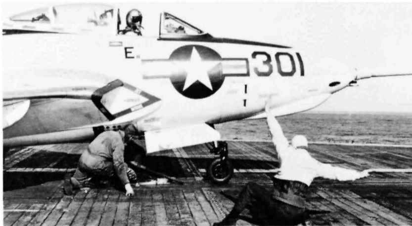
F9F-8 Cougar being secured for catapulting (RAF Museum)
