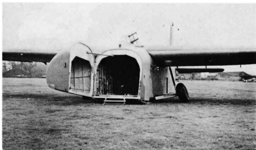
Hamilcar's collapsing undercarriage and large nose door
