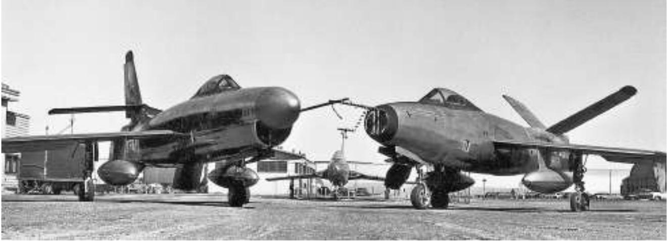
**Above: The two XF-91 prototypes, 46-680 on the left, in its final configuration with a radome fitted to the nose, above a modified chin-type intake. On the right is 46-681, now fitted with a 'butterfly' tail. Between them, in the background, is the YRF-84F Thunderflash prototype**
